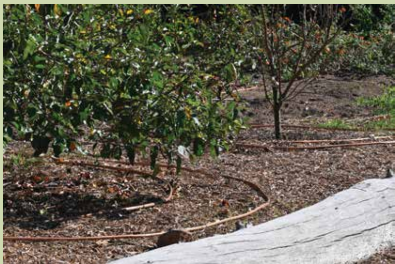
Newly installed anti-intrusion copper drip tubing prior to being covered with mulch.
