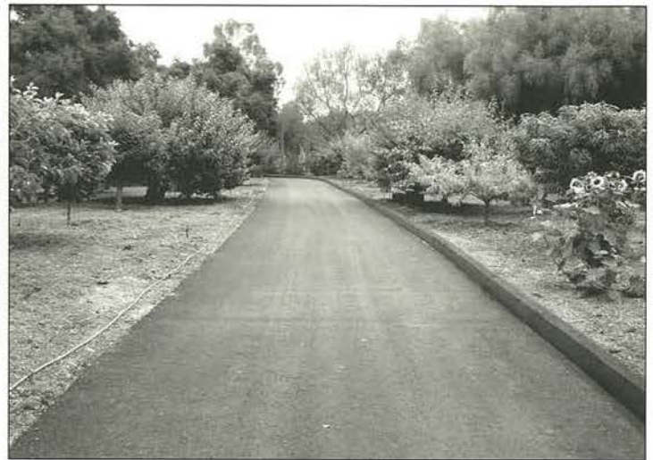
A 2 percent grade toward the six-inch curb channels storm runoff away from landscaped areas.
